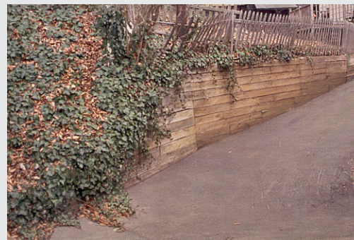
A relatively recent retaining wall constructed with wood beams. (The visual appearance of this wall could be improved by planting and allowing vines to grow up and cover it.)
