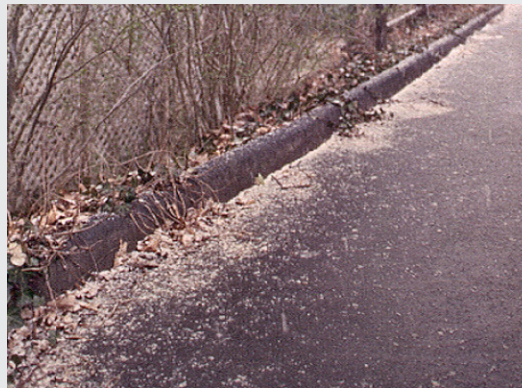
(Above) Rolled asphalt curbing was installed on the upper parts of Cherokee and Canterbury Roads.
