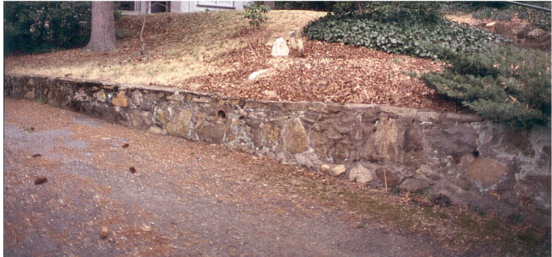
The primary form of wall used in Albemarle Park is the low stone retaining wall, rarely exceeding 3' in height. It is used to effect a change in grade where an unsupported
