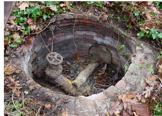
(Above) Steam valve in a brick-lined pit behind Manzanita Cottage. This controlled the steam heat coming from the Manor Inn's boiler to several of the cottages up the hill.
