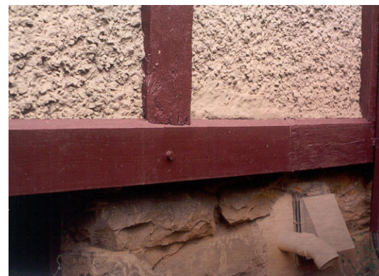
Below: Close up photo of the new stucco and band board, applied with care, to restore the original appearance of the wall.
