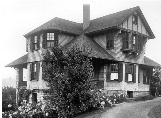
Clematis Cottage possesses many of the design features of this style - half-timbering in the gables, shingles at the 2nd floor; pebbledash stucco at the 1st floor, and a stone foundation.
