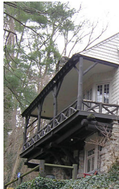
Below left: Porch at Crow's Nest, made from large timbers stripped of their bark.
