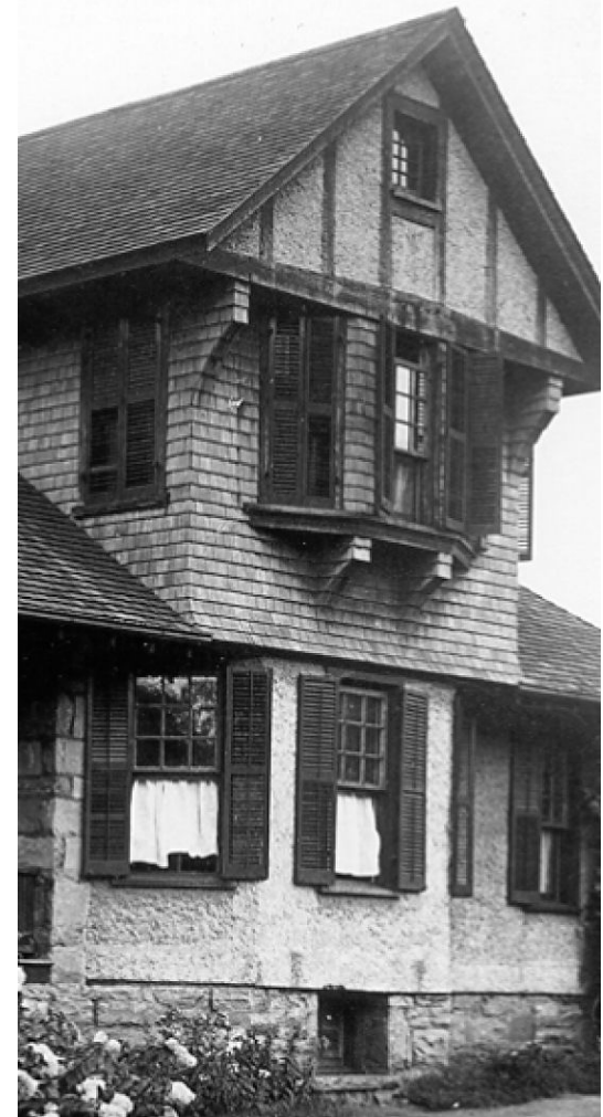
Clematis Cottage possesses many of the design features of this style - half-timbering in the gables, shingles at the 2nd floor; pebbledash stucco at the 1st floor, and a stone foundation.
