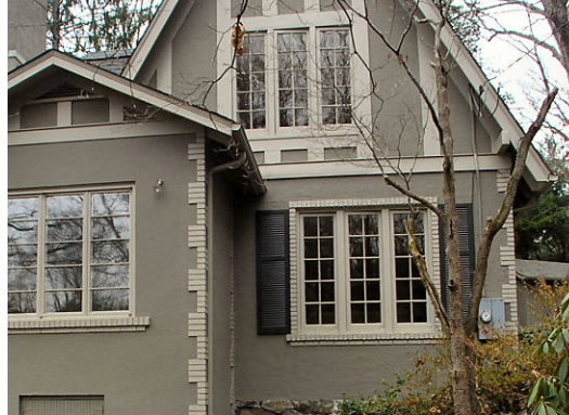
Above: Signature details of architect Richard Sharp Smith on Chipmunk Cottage - brick quoining at the corners, brick window sills and surrounds, half-timbering in the 2nd floor, and smooth stucco exterior finish.
