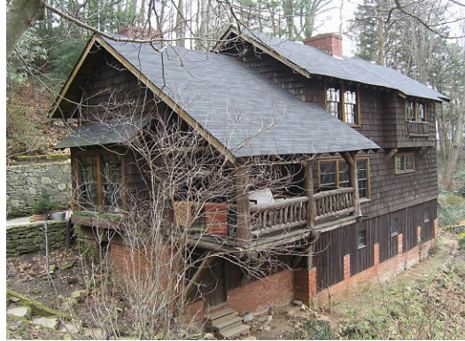
Above: Possum Trot, displaying several of the key elements of the Rustic Shingle Style - dark brown stained shingles, large timbers used for porch supports, and projecting bay windows.
