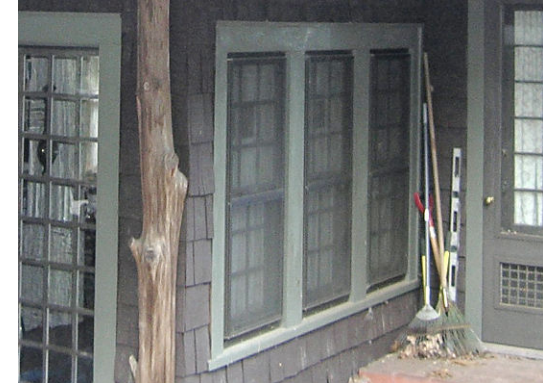
Above: The exterior storms on these windows are full-screen, painted the same color as the windows sashes, with the cross-brace at the same height as the meeting rail of the two window sashes.
